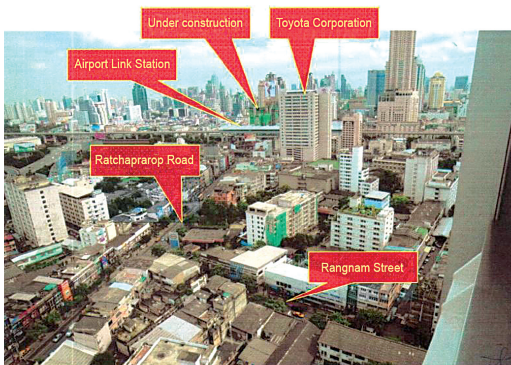
Picture 17: This site investigation picture from the Institute of Forensic Science shows the area on the left side of the Metropolitan Gypsum building. It was taken from the balcony where the incident described in point 2.3.10.5 (2) took place. 249
